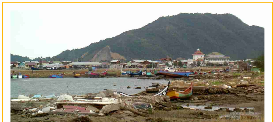
The impact of the 2004 tsunami remains visible even after three years.
