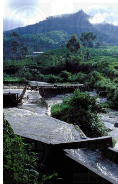
Canals channelling water to mini hydroelectric plant
