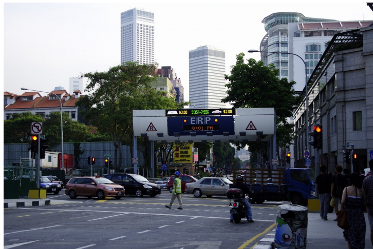
Singapore's Electronic Road Pricing (ERP) system was one of its early initiatives which leveraged on information technology to manage road congestion.
