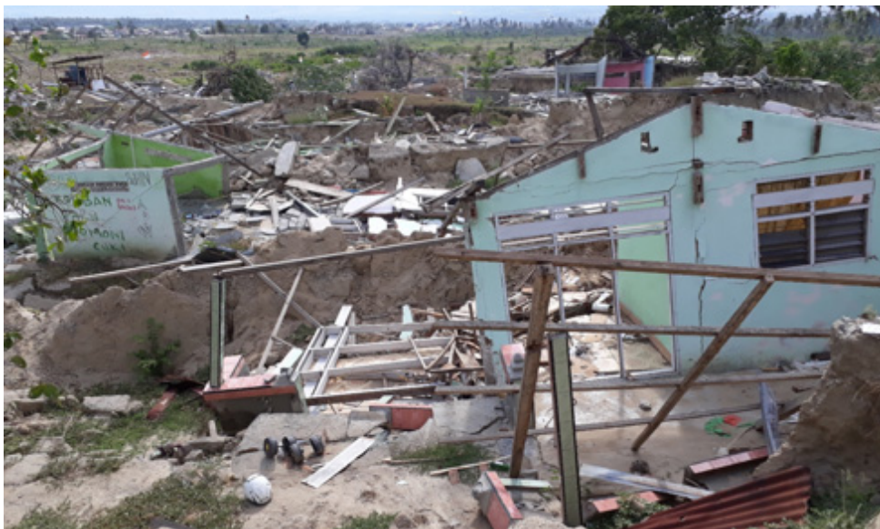
Remains of houses in Petobo devastated by landslides and liquefaction.
